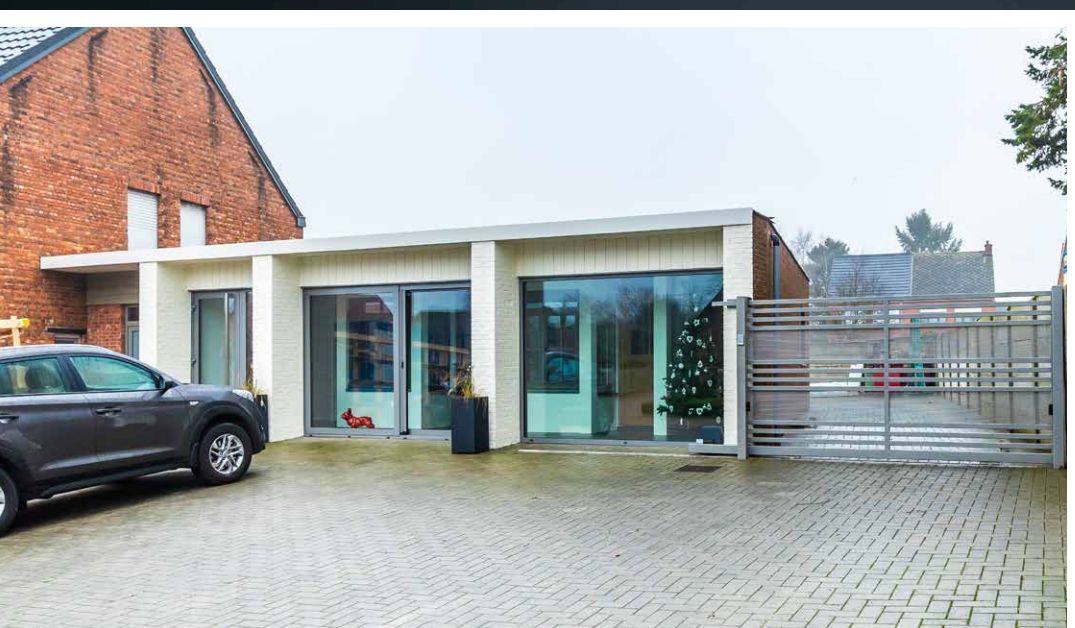
PEKO CONSTRUCT - Reynaers Installer in Meerhout
